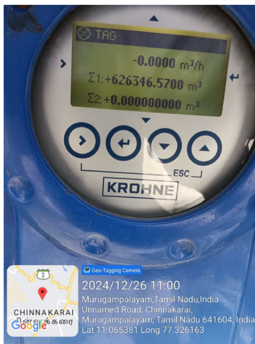
Flow Meter – Outlet (RO Permeate to Member Unit)
